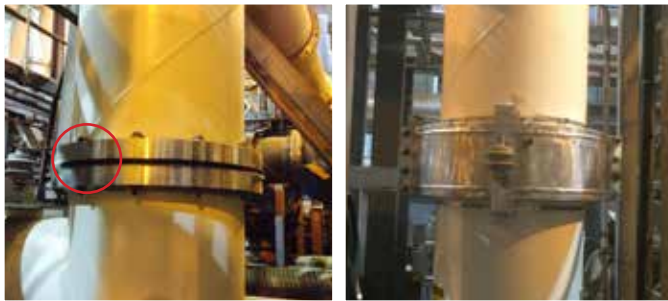
Above left: A leaking flange at Southern California Edison's Valley GIS. Above right: the installed custom enclosure from Colt.
