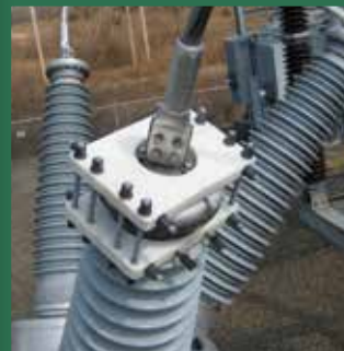
Above left: A leaking flange at Southern California Edison's Valley GIS. Above right: the installed custom enclosure from Colt.
