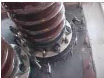
Leaking Bushing Repaired
