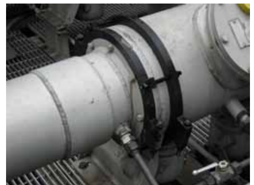
Gas insulated buss flange repaired on-line.
