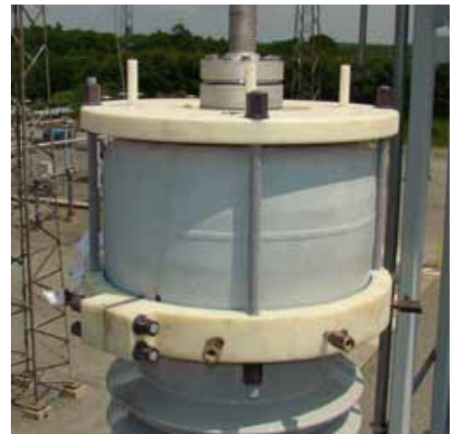
A bushing flange with a custom repair clamp installed and sealed.
